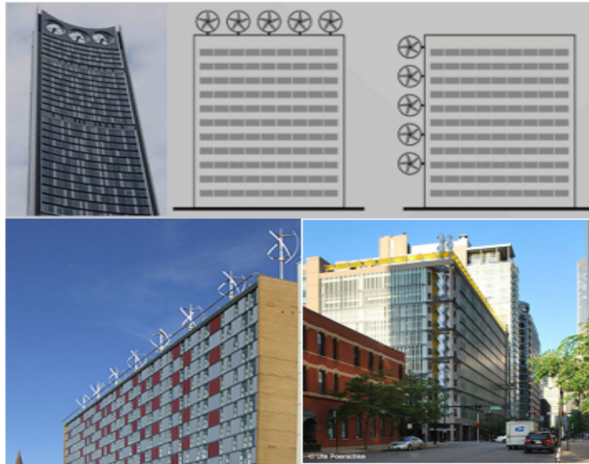
Figure 3. Building Integrated Wind Power System[7][15]
