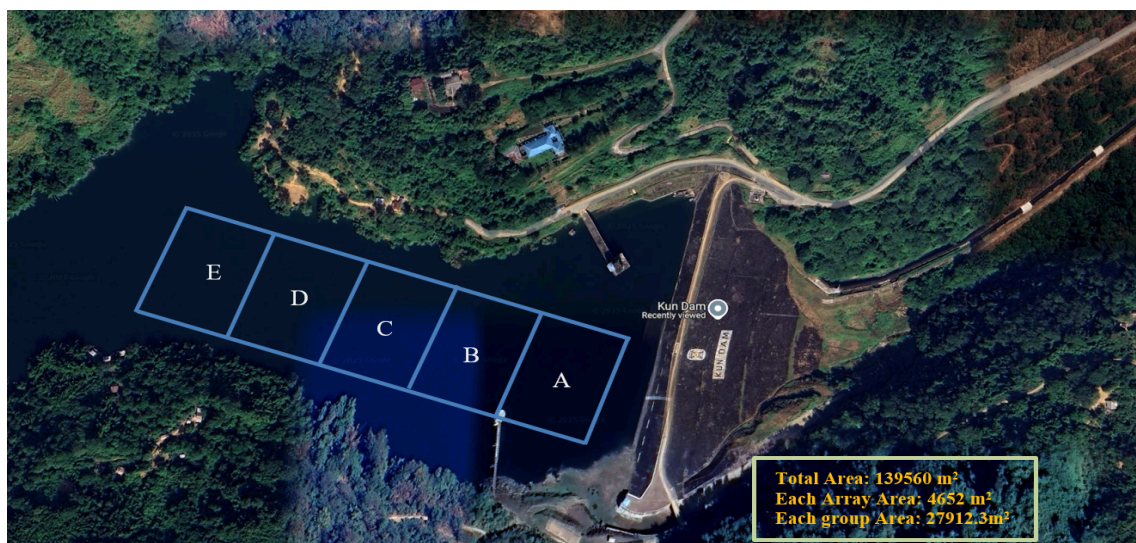
Figure 2. Installed PV System Area on Kun Chaung Dam
