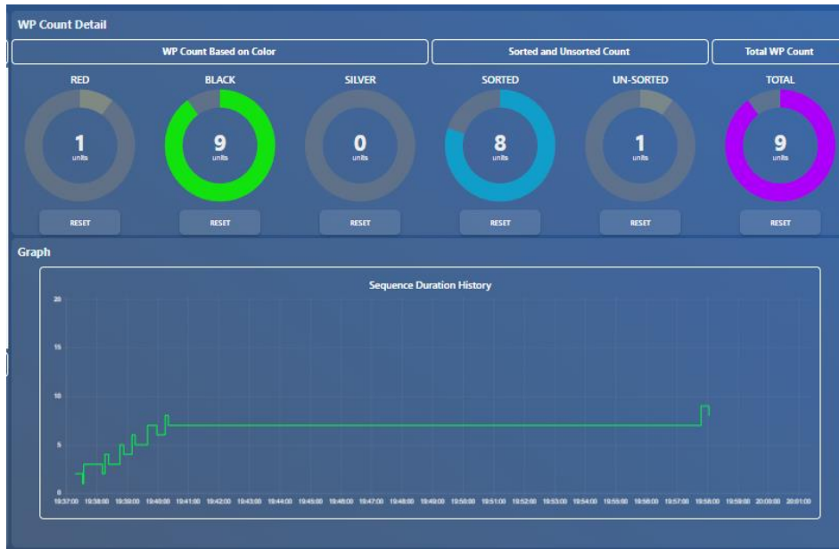
Gambar 6. Tampilan SCADA Separating Station 2
